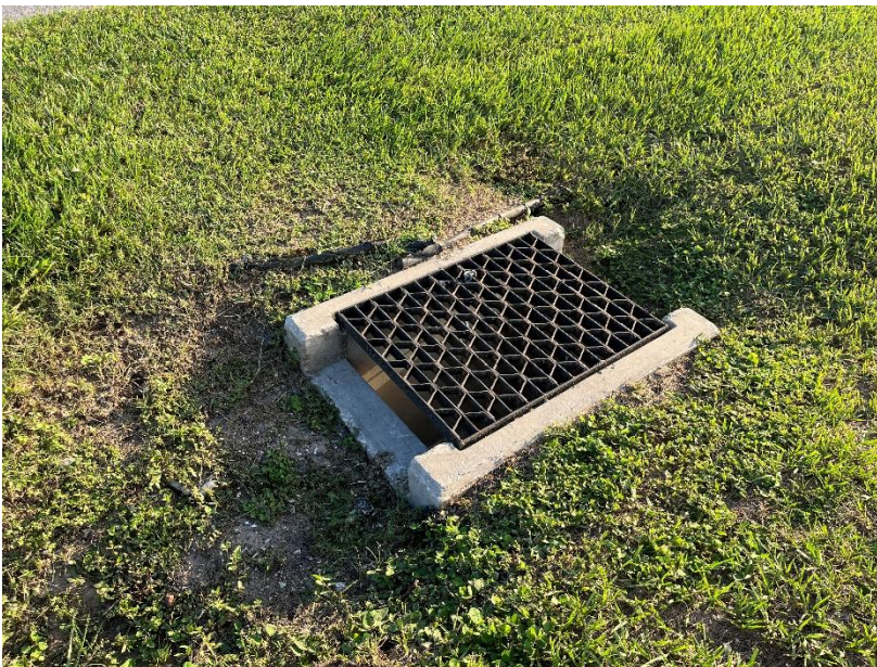
Figure 4. Grate inlet in good condition
