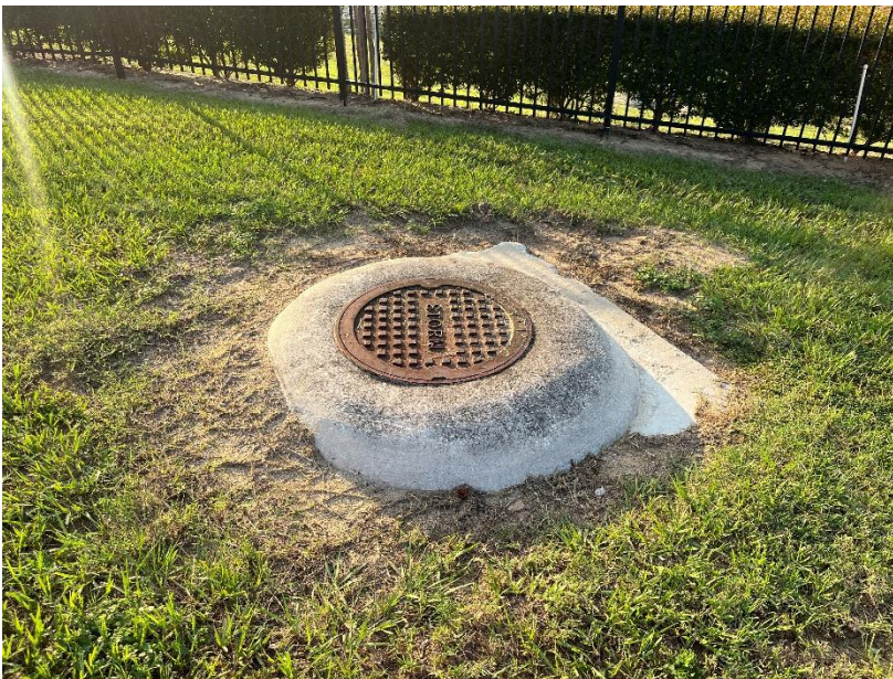
Figure 6. Manhole in good condition.
