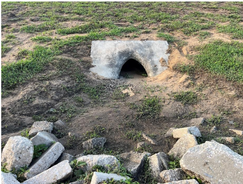
Figure 10. End section in poor condition., Monitor clearing of sediment.
