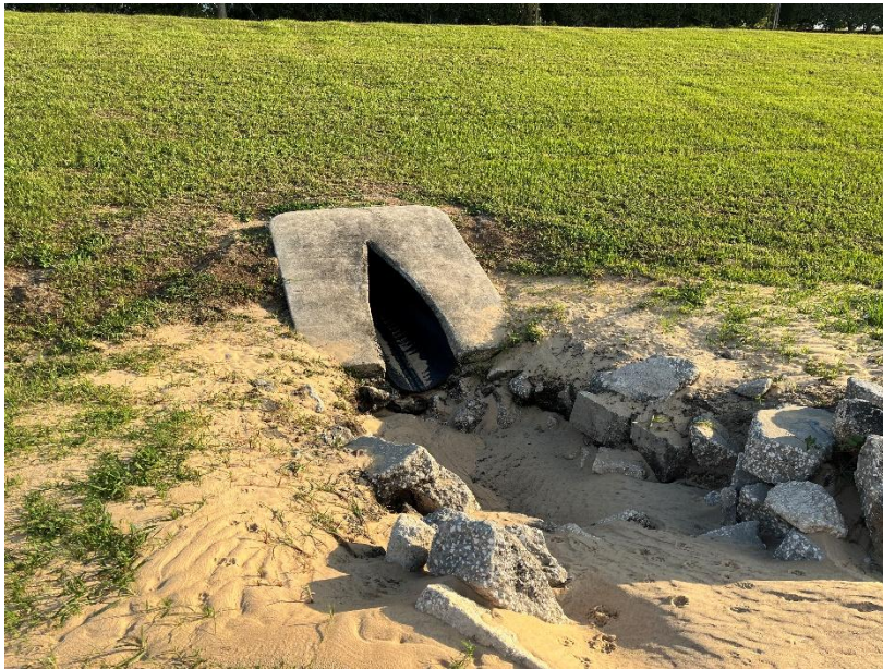
Figure 2. End section in good condition.
