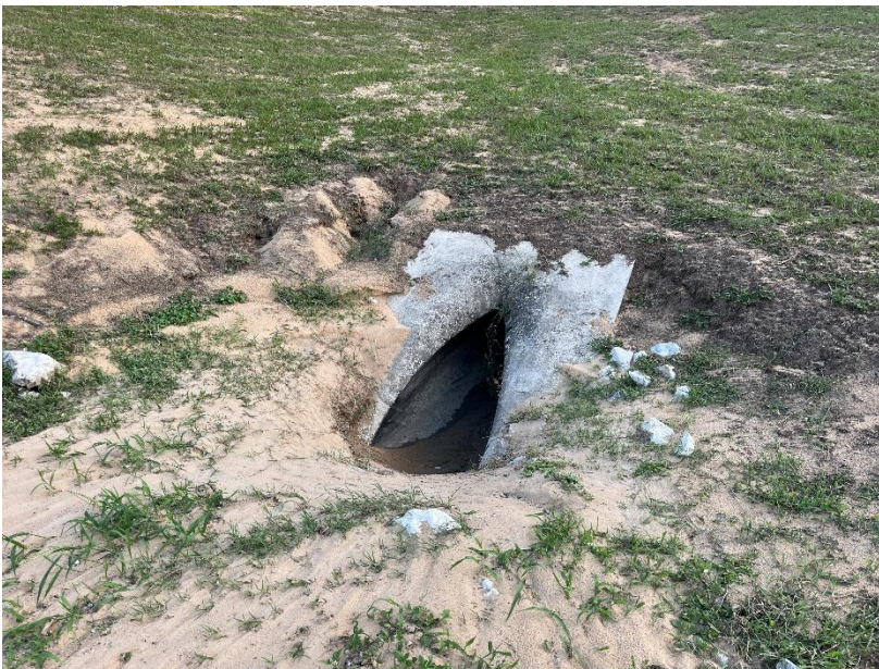
Figure 8. End section in fair condition. Monitor clearing of sediment.
