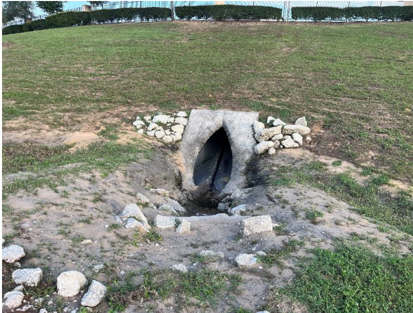
Figure 10. End section in poor condition., Monitor clearing of sediment.
