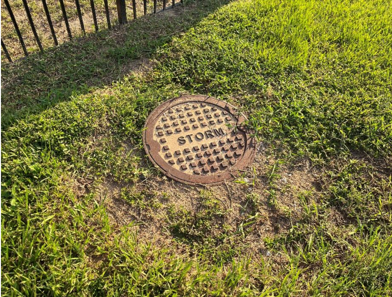
Figure 6. Manhole in good condition.
