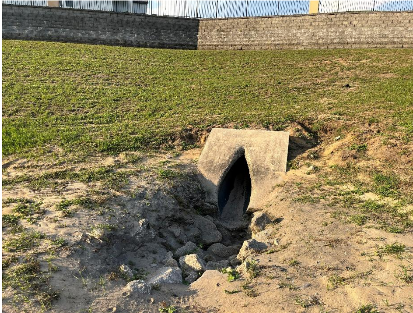
Figure 2. End section in good condition.
